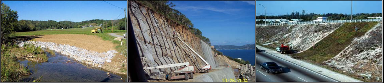
Bank Stabilization – adding materials to a bank to prevent erosion
