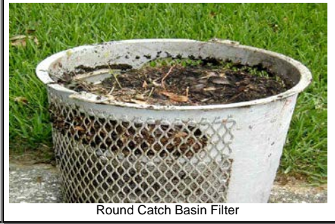
Water flows into the removable basket, filtering trash, leaves, yard clippings, sediment, etc.
