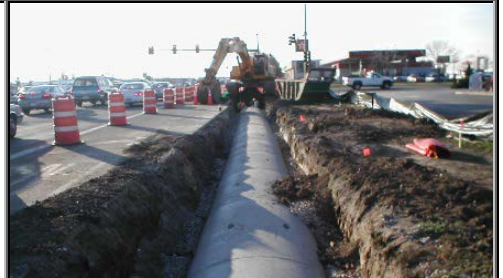
HDPE – High Density Polyethylene Pipe
