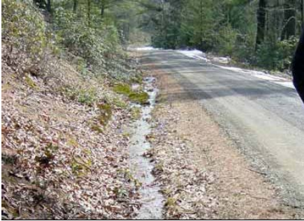
The ditch above carries water from roadside springs. An underdrain can collect this flow to keep the roadbed and ditch dry.
