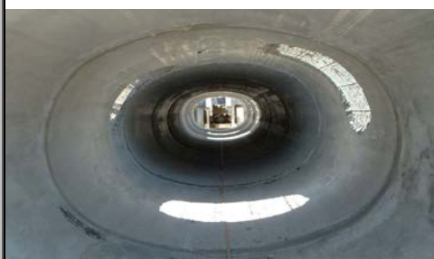
HERCP – Horizontal Elliptical Reinforced Pipe
