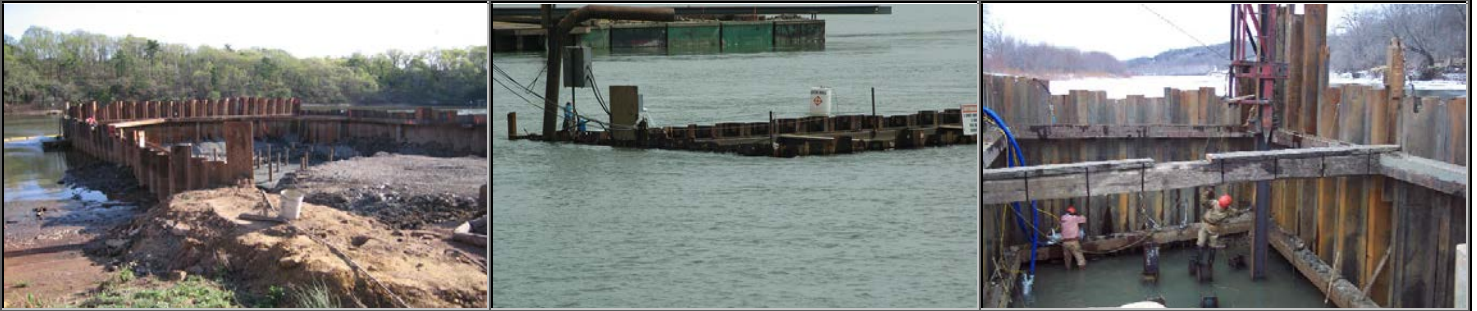
Cofferdam, Sheet Pile
