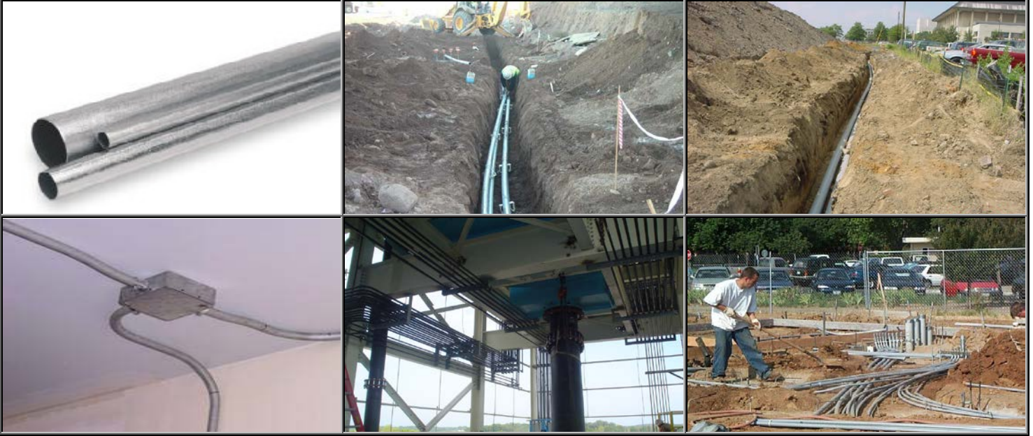
Conduit – a pipe system used to protect cables.
