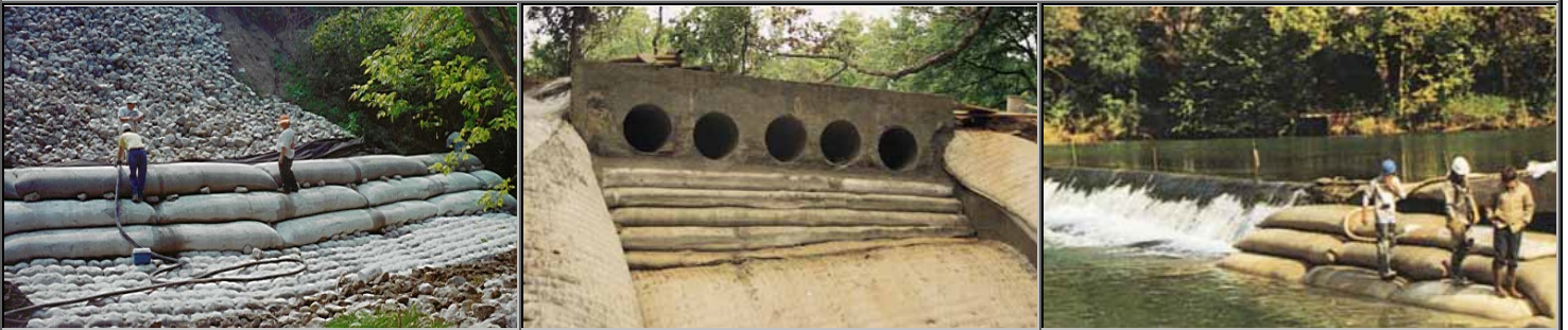
Concrete Bags – riprap alternative.
