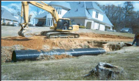
Construction of culvert
