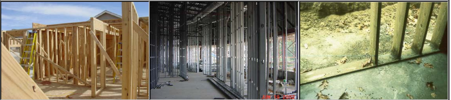
Studs, Wall – a vertical member in light frame construction.
