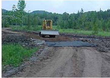
Geotextile creates stable road base
